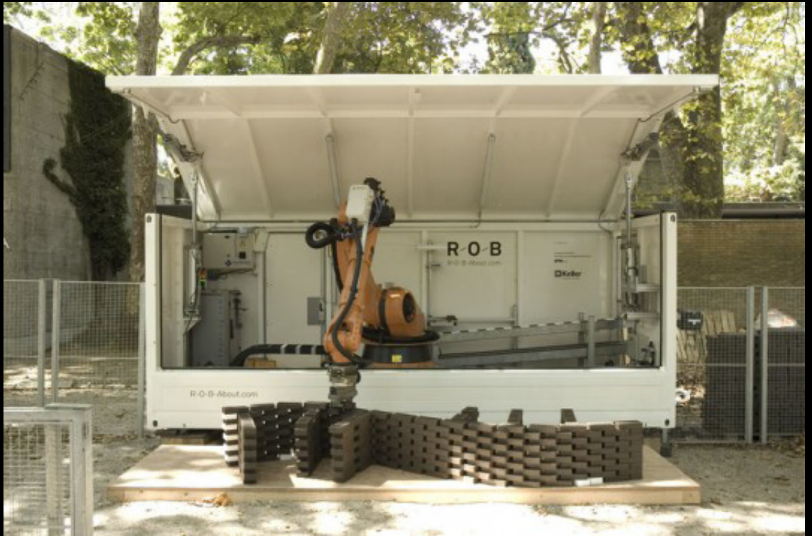
Robot Employed On Site
